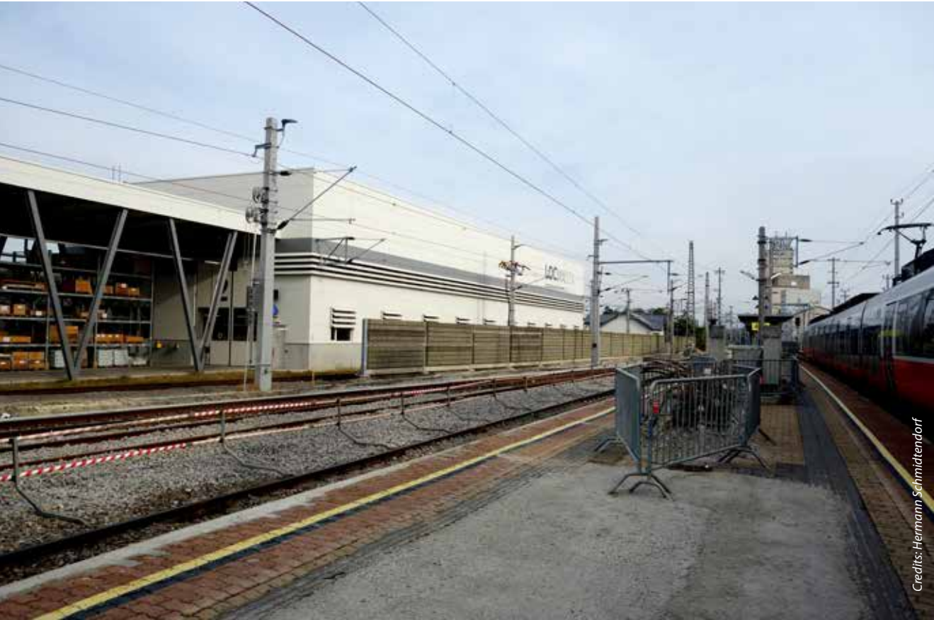
The LOCMASTA workshop building is on the left in the picture. The tracks continue towards the Hungarian border on the horizon.
