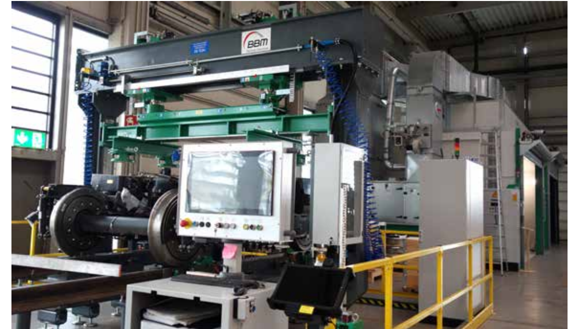
Gersthofen: a complete production line for wheelset replacement and machining, spring pressure stands and painting systems
