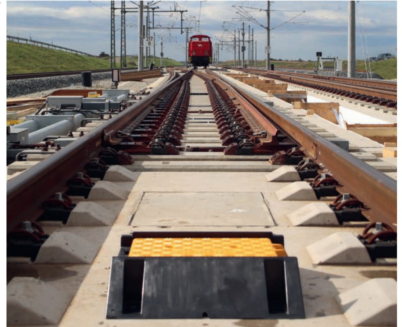
Working together for new rail technology: Siemens Mobility and Leonhard Weiß. The photo shows the new line "German Unity Transport Project No. 8."
