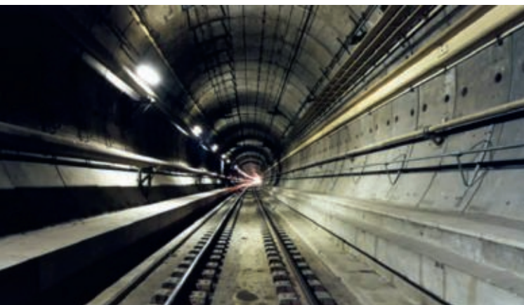
Extremely stable: View into a tube of the Eurotunnel.
