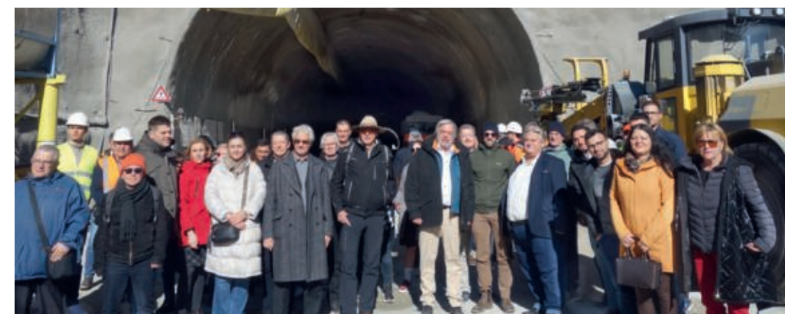
At the railway construction site Sofia-Plovdiv.
