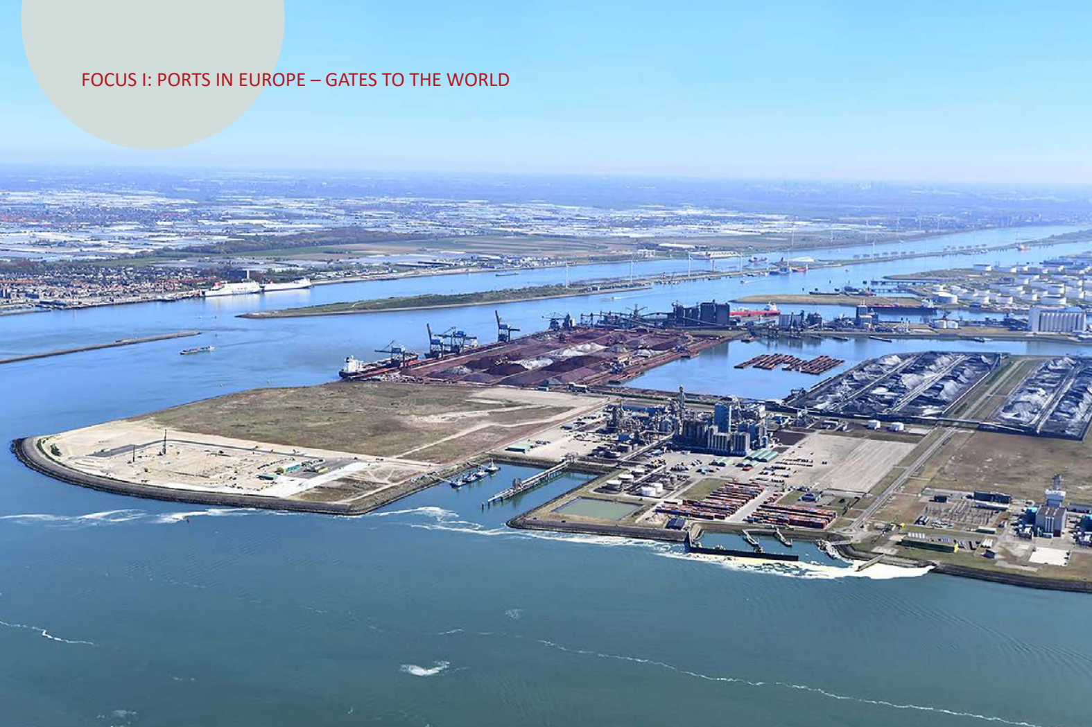
The port of Rotterdam continues to grow – here on the construction site Kop van de Beer.
