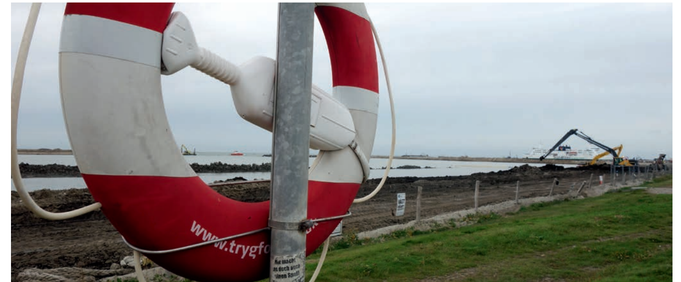
Work is in full swing in Rødby.
