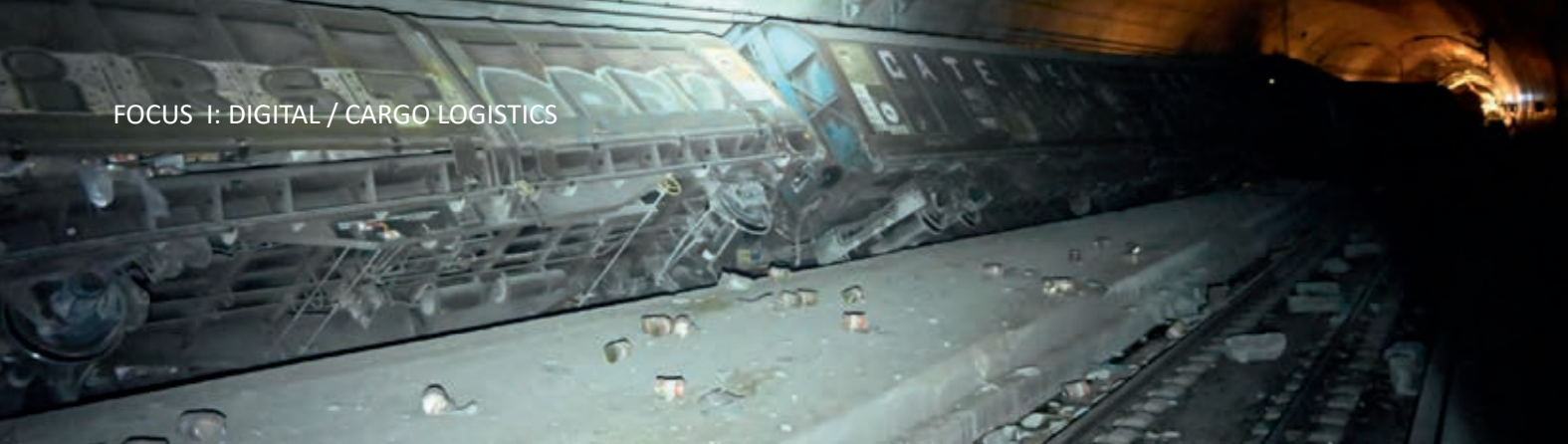
A single broken wheel, but major damage: The derailed train in the Gotthard Tunnel.
