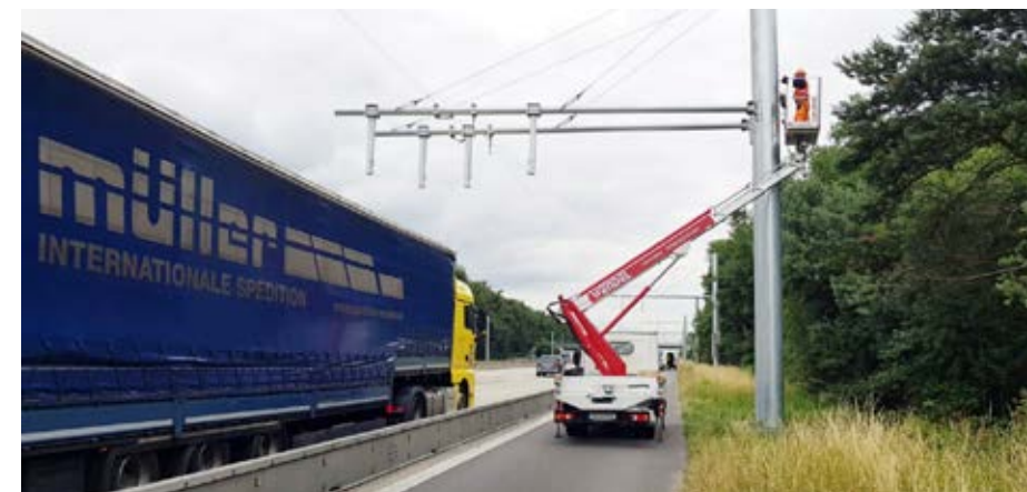
Autobahn A5 Darmstadt – Frankfurt am Main
