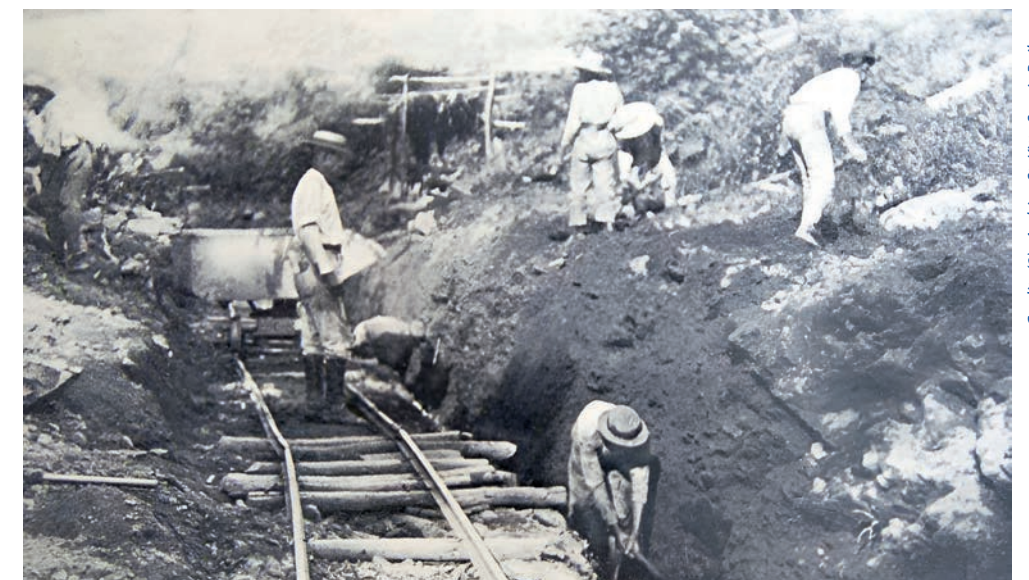
During the construction of the sugar railway in 1912.
